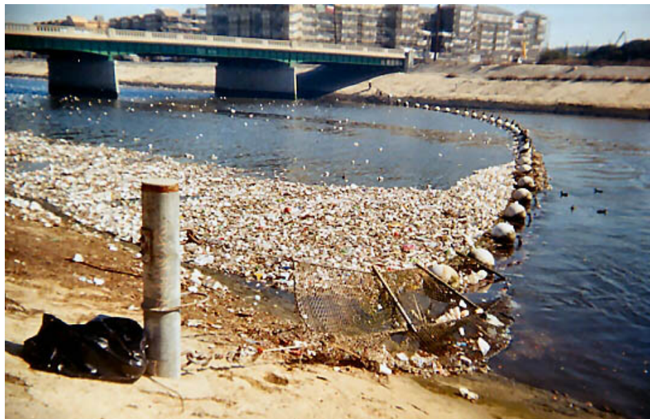
The trash net on Ballona Creek at Lincoln Blvd captures trash after a rain, but during heavy storms, the net is removed because the volume of water is too great.
