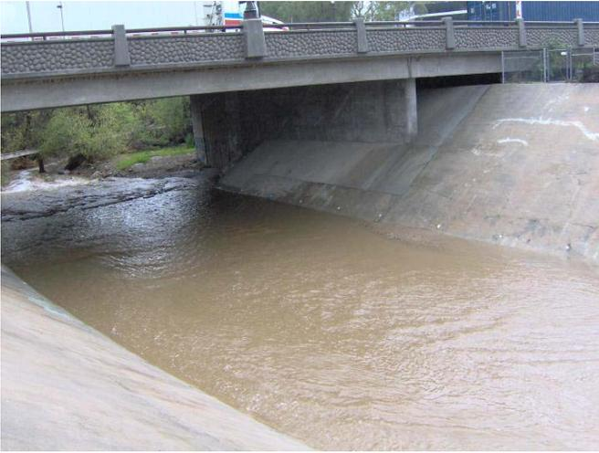
One consequence of removal of the natural stream bottom and riparian vegetation was to prevent some species (fish and perhaps some amphibians and small invertebrates which burrow in the mud) from crossing that 400-foot stretch. Another was "thermal pollution", in which the concrete channel bottom warmed the inch of water above it, increasing the heavy algae blooms that also infest Ballona Creek in warm weather. The 400 feet became a barren and ugly zone.
