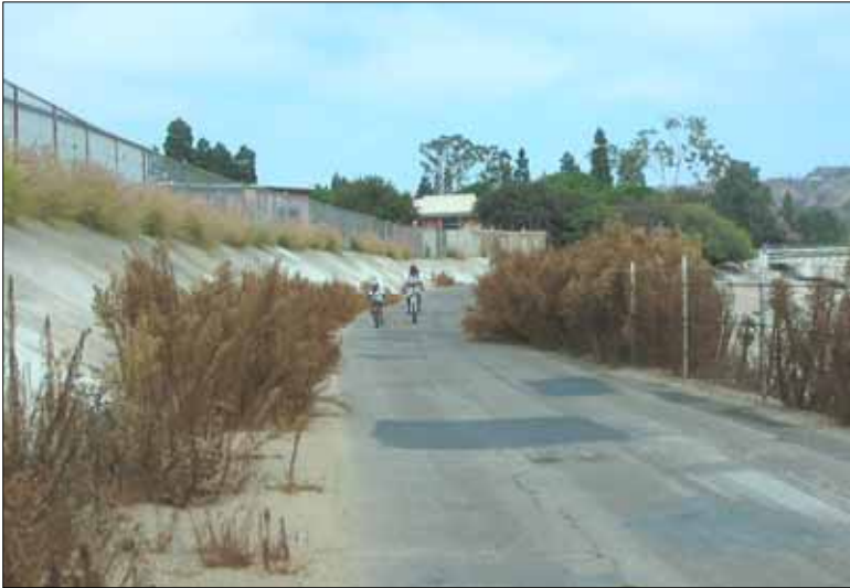
Left: Looking east along the Culver City section being renovated between Overland Ave. and the pedestrian bridge, showing cracked blacktop, concrete-sprayed slopes, and giant weeds. Right: artist's conception of same section after renovation.
