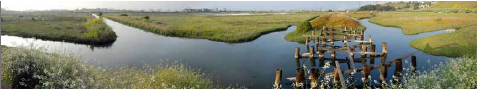
Tidal channels and old Pacific Railway structure in area B. (Photo by Jim Everett)
