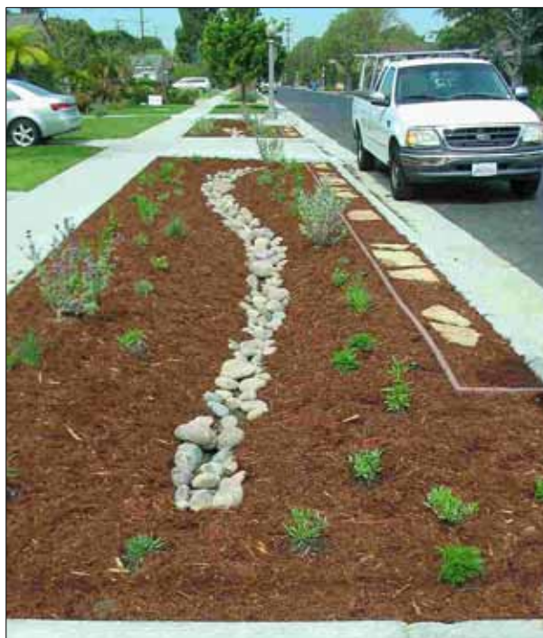
Left: construction photo by Culver City Public Works
