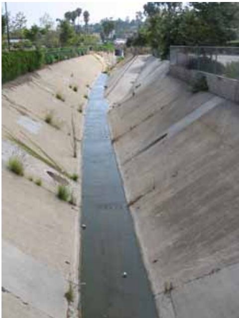
Buena Vista Creek looking upstream...
