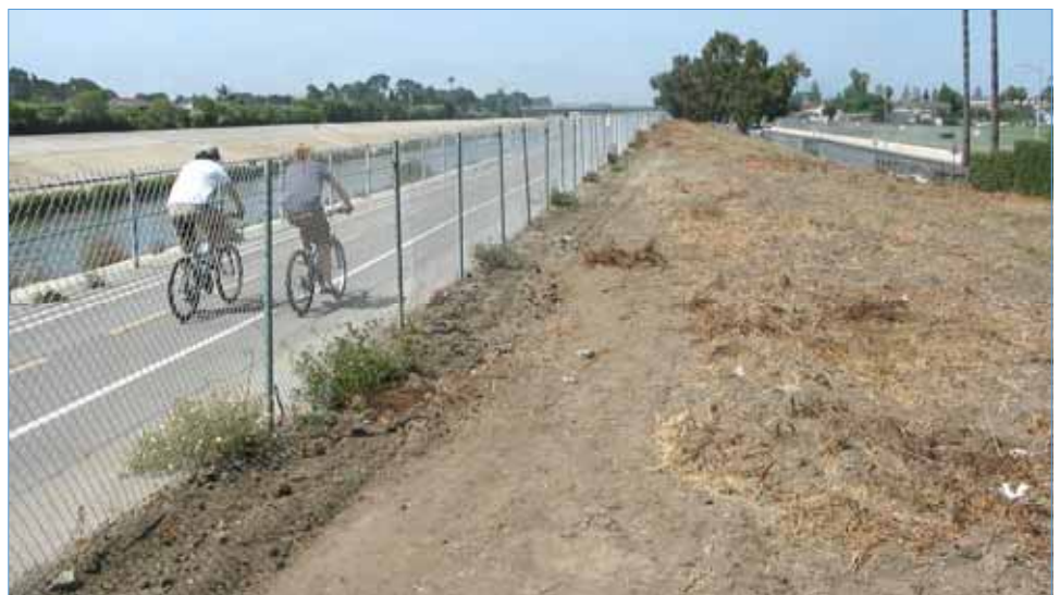
The Milton Street parcel before construction, looking west, with the creek and bikepath on the left and Milton Street and a corner of the Marina del Rey Middle School athletic field on the right
